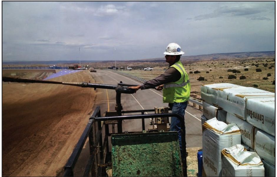
The concentrated compost soil amendment was hydraulically applied by the contractor, 814 Solutions. This method allows for extended reach and a uniform coverage.
