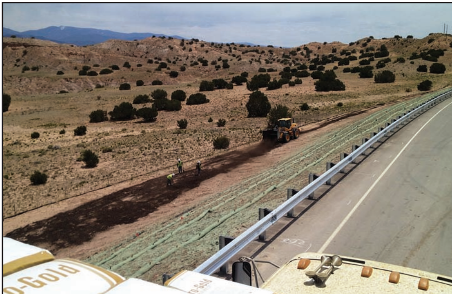
Three laborers and an equipment operator were required to apply the NM DOT compost.
